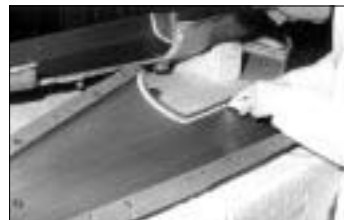
Filled resins being applied with brush and piping bag
